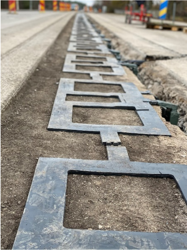
Coils under the road
